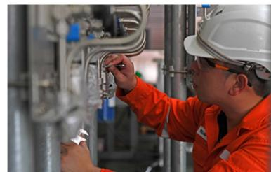
**FIG. 3.** The best installation practices include using a gap inspection tool to verify fittings are tightened properly.
