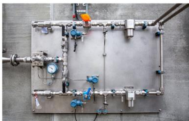
**FIG. 2.** The fluid systems that supply water to the electrolyzer and capture the resultant H<sub>2</sub> and oxygen gases are central to determining how well an electrolyzer will function.
